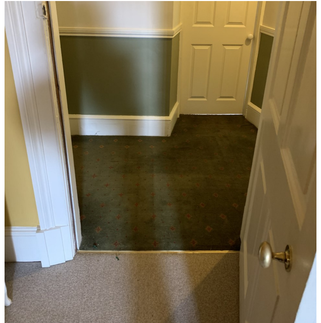
Flat entrance into rooms
