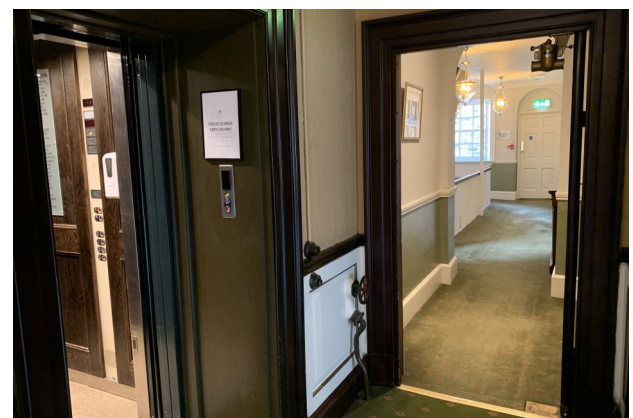
The lift on the ground floor leading to outside
